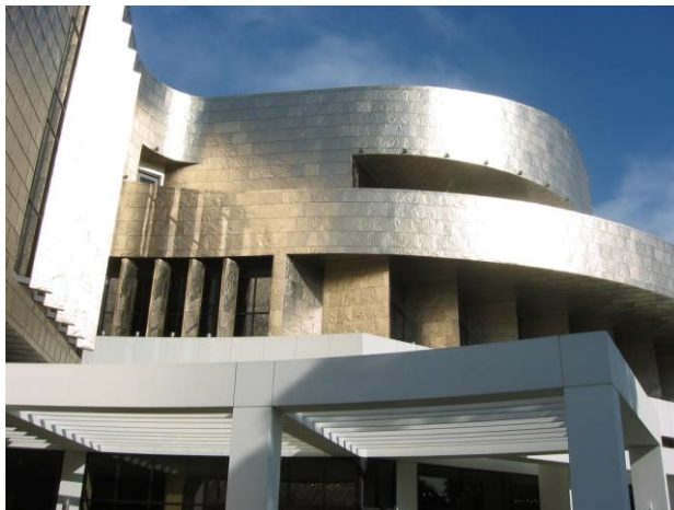
Fig. 2. Cerritos Library, California. The new portion of the building is clad in titanium, the first building in the U.S. to use this material. It shimmers in the light and changes color with the weather.
