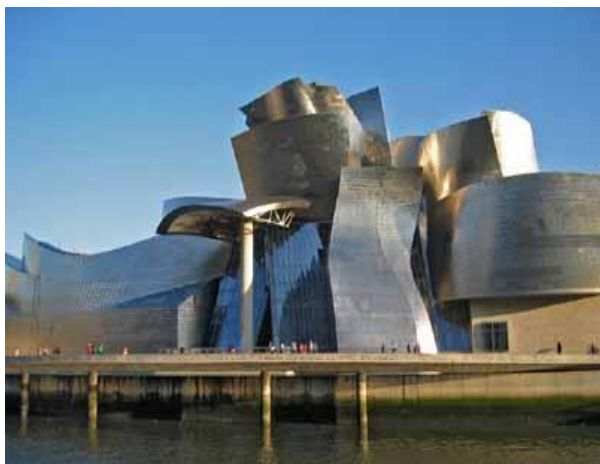
Fig.1. Guggenheim museum Bilbao, Spain
