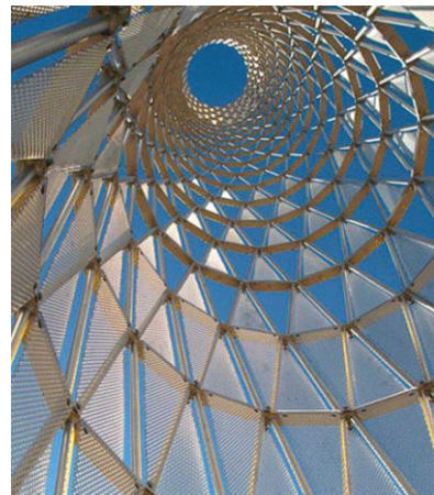
Fig. 18. UNMC Tower with gold-tinted Ti
